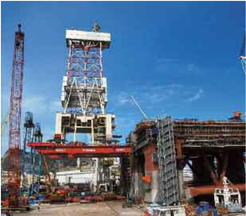
[Figure 8.5 – Drilling Tower Module lifting and skidding with elevator system for Scarabeo 8 Saipem Platform in Fincantieri Palermo (Fagioli)]
