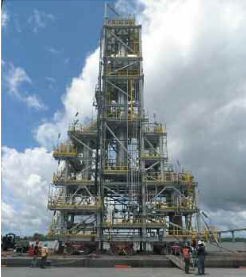
[Figure 9.8 – Load out project of a module]
