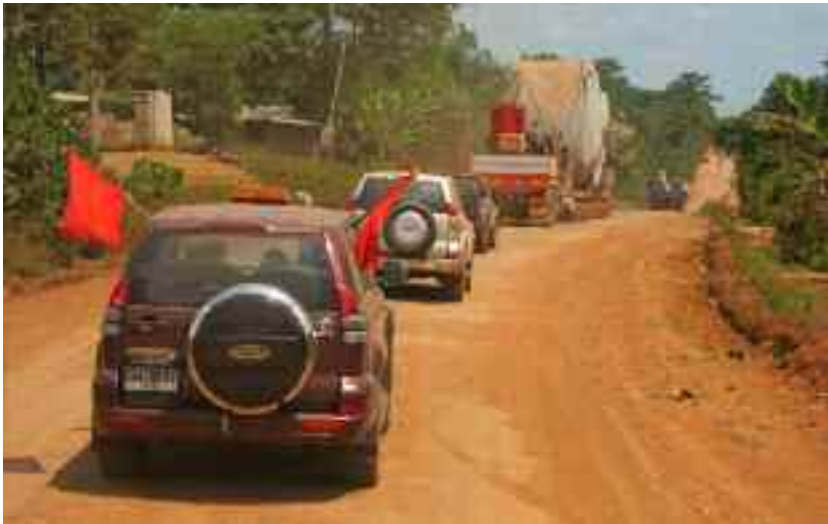
[Figure 4.11 – Site Survey]
