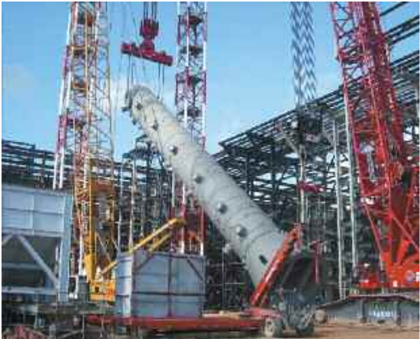
[Figure 5.2 – Reactor lifting for Saipem GNL 3Z Project Algeria (Fagioli)]
