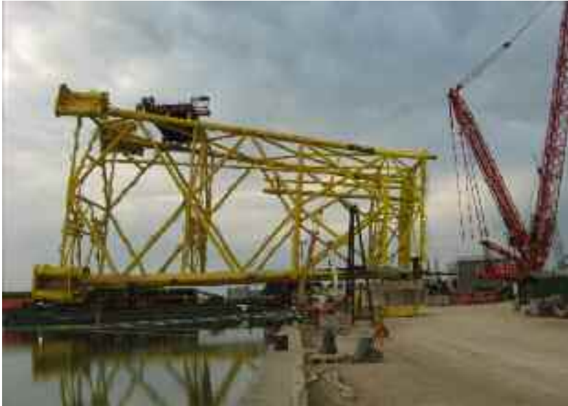
[Figure 10.2 – Jasmine Jacket load out by skidding operation in Rosetti]
