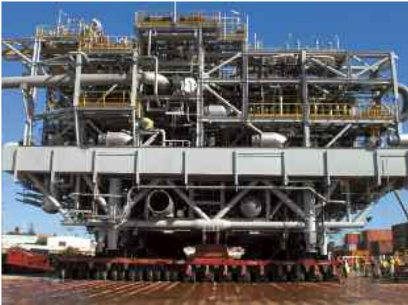
[Figure 10.4 – Load out project of a module]
