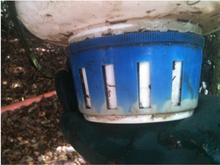
**Figure 1.** Opening the chlorinator.
