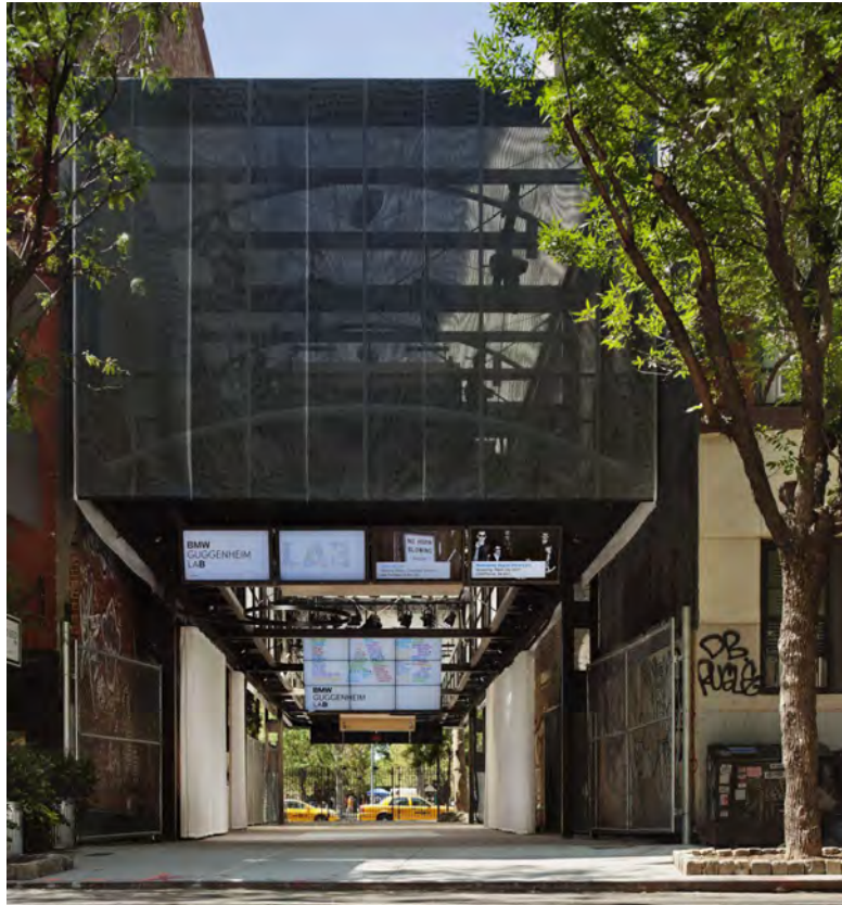
IMG. 5.07 — Exterior view from East First Street of the BMW Guggenheim Lab, New York City, USA. Project by Atelier Bow-Wow from Tokyo: the structure is designed to be responsive to the cities that the Lab visits. © Solomon R. Guggenheim Foundation, New York. Photo by Paul Warchol.
