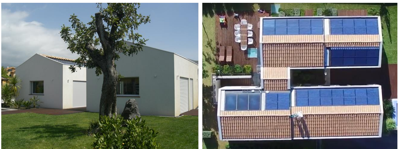
Fig. 1. External (left) and aerial (right) view of the building.
