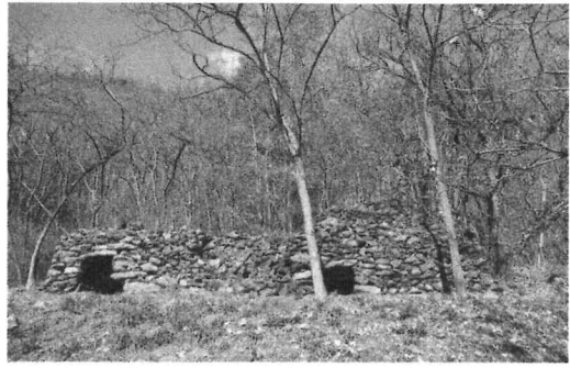
Figure 3. Small constructions built entirely with dry stone, with circular base and false-dome covering, locally named baitelli .
