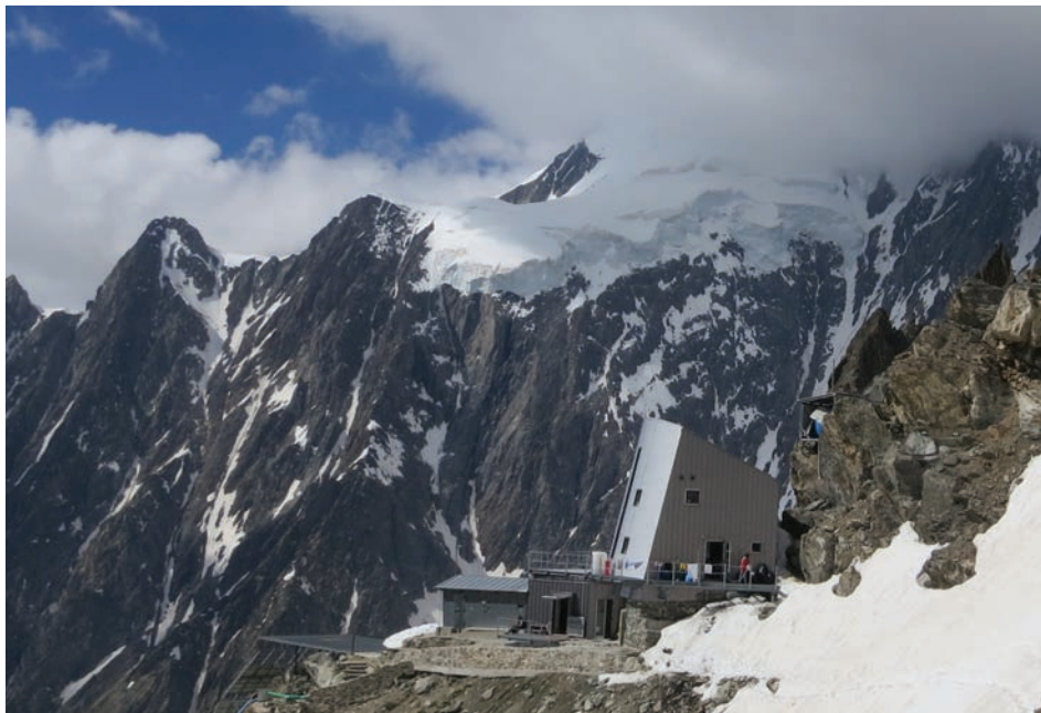
Figg. 8-9. Gonella hut , Courmayeur. State of the art before and after reconstruction, 2016. Photo by Roberto Dini
