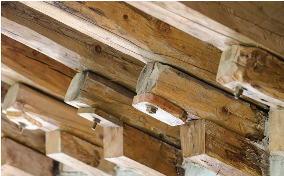
Fig. 5. Detail of the roofing. Photo by Alpes/Giorgio Dalvit ©
