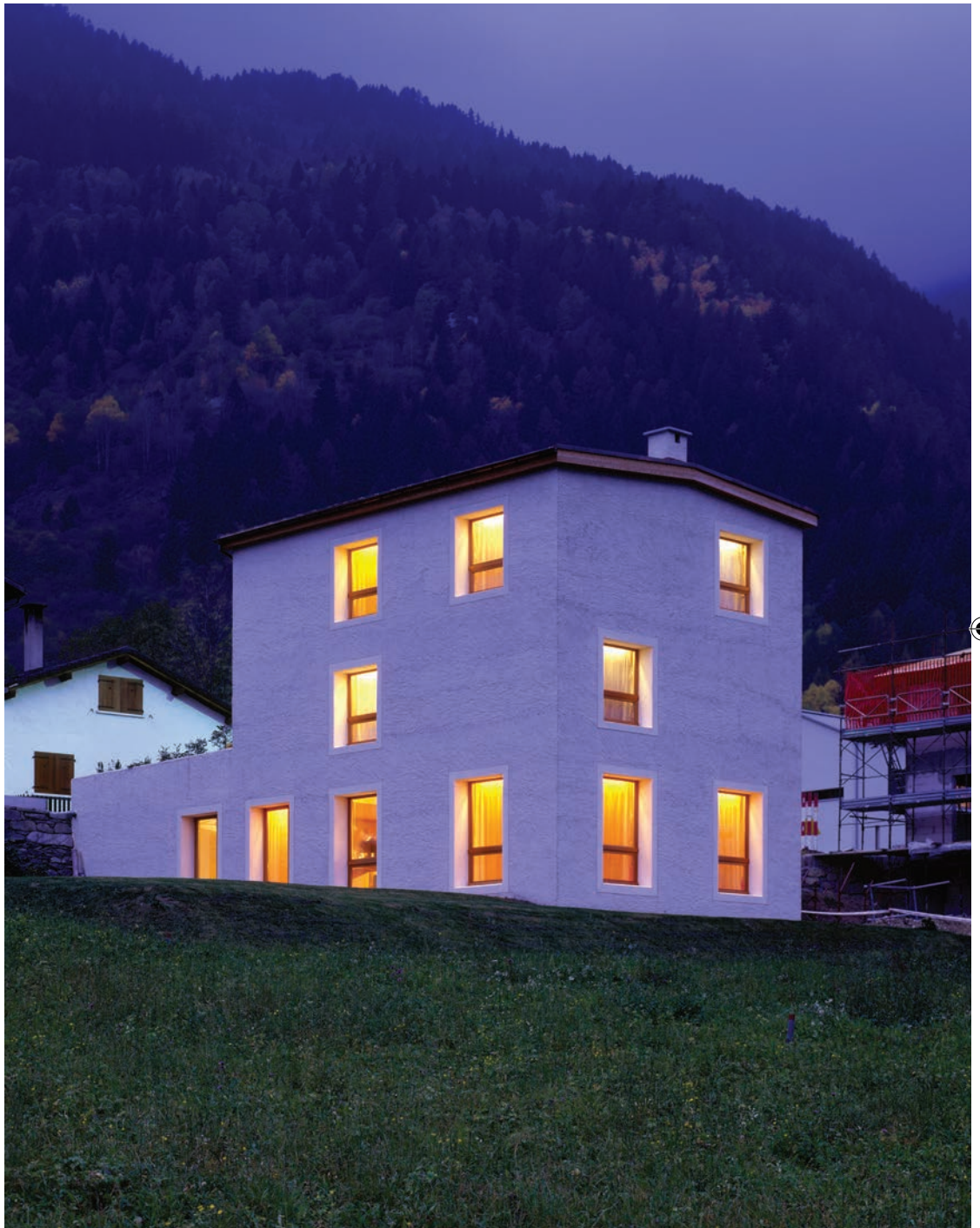
Fig. 7. Raselli House in Poschiavo, Grisons, 2001-2002. Photo by Ralph Feiner ©
