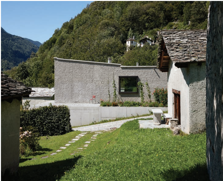
Fig. 5. House in Castasegna, East Front. Photo by Ralph Feiner ©
