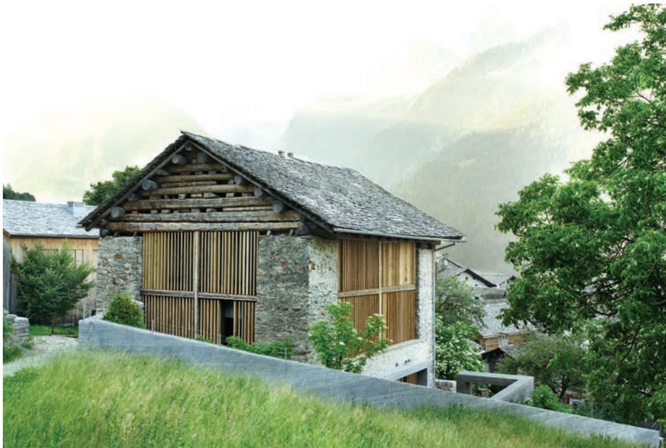
Fig. 8. Recovery of a disused stable in Soglio, after renovation
