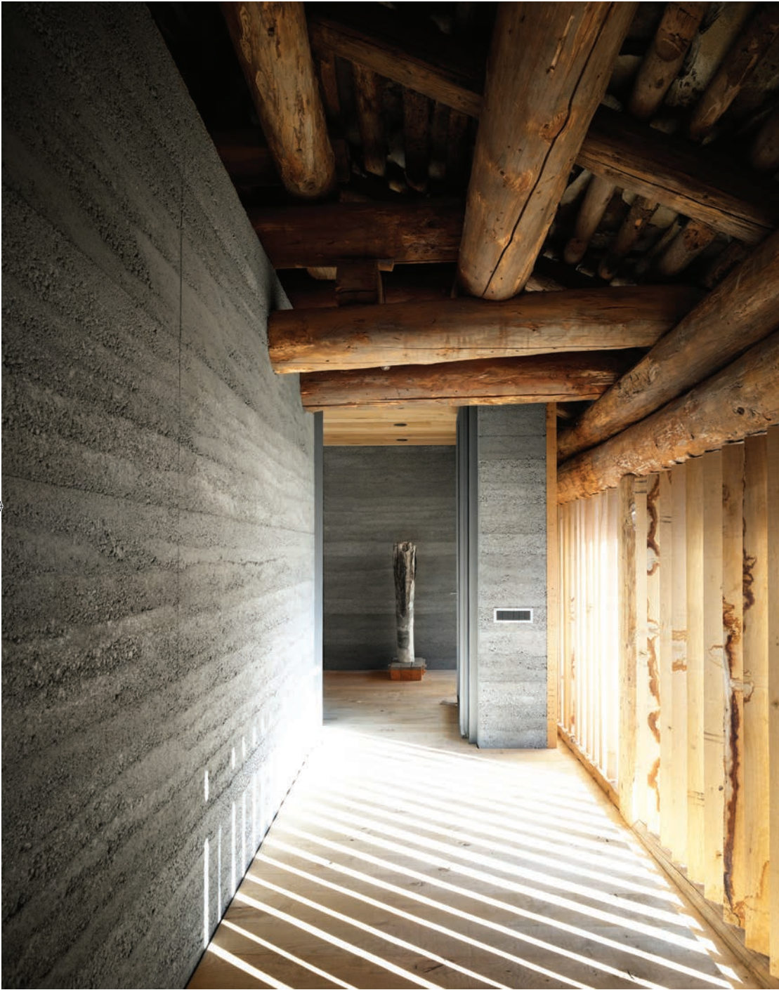
Fig. 11. Recovery of a disused stable in Soglio, loggia entrance
