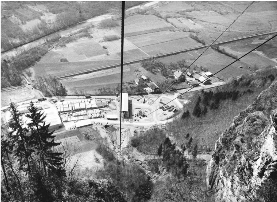
Fig. 8. The cableway and the prefabrication yard in the valley floor. Centre culturel de Flaine ©
