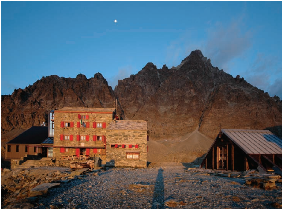
Fig. 4-5-6. Quintino Sella hut at Monviso: the original central nucleus (designed by Ubaldo Valbusa, 1905) has been repeatedly expanded and renovated (in particular in 1998-2001, on Gian Mario Bertarione's project)
