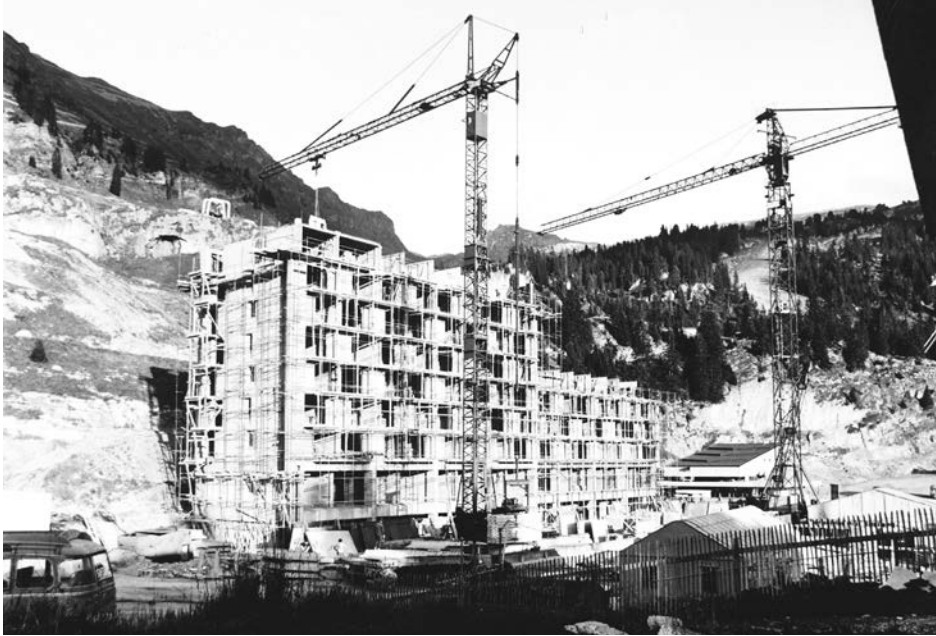
Fig. 7. Construction process of the Aldébaran building . Centre culturel de Flaine ©
