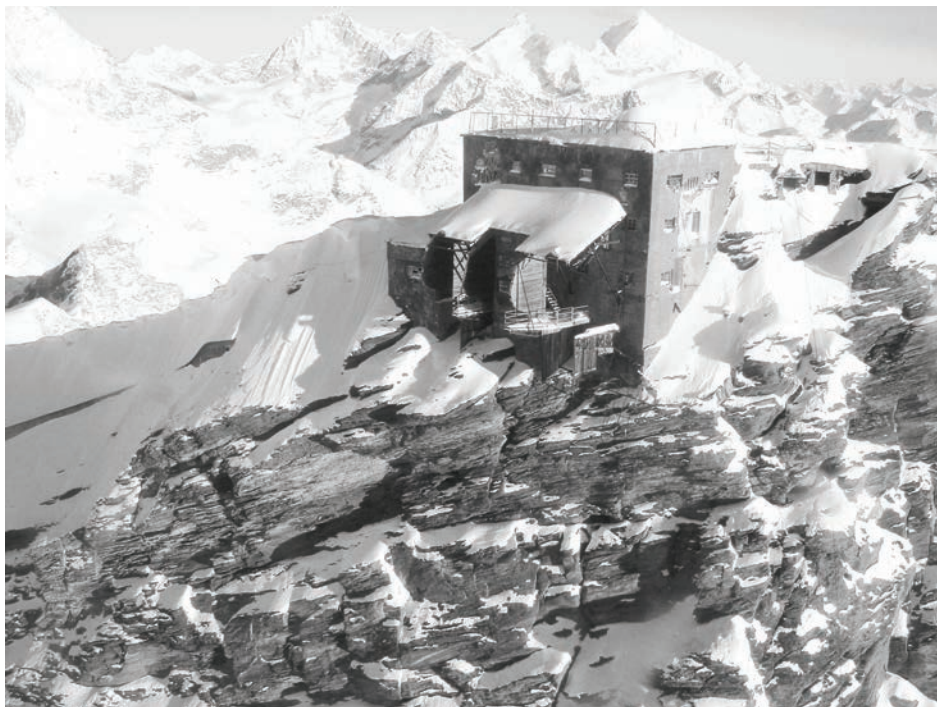
Fig. 2. The abandoned Furggen's cableway arrival station
