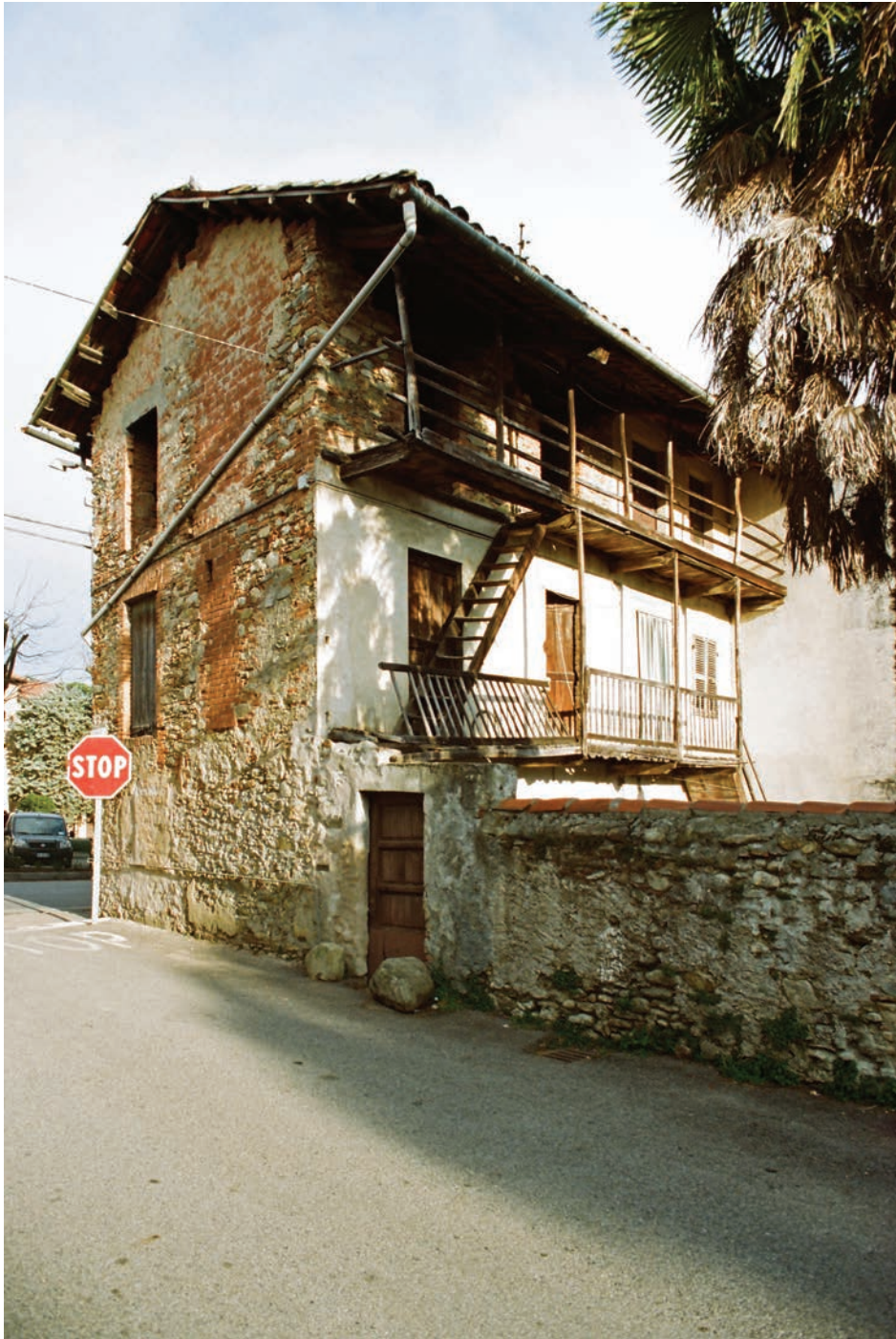
Fig. 6. Rural House. Rivara Canavese
