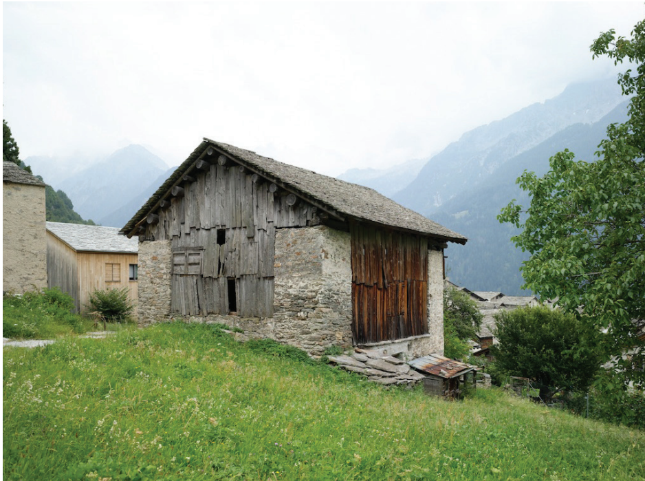
Fig. 7. Recovery of a disused stable in Soglio, before renovation
