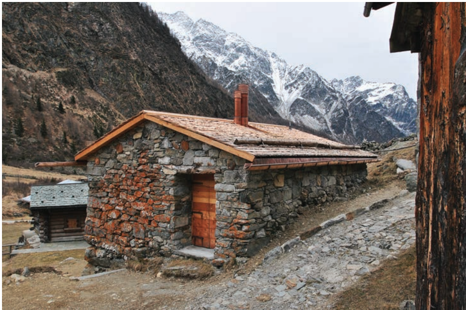
Fig. 3-4. Stone house in Val di Rezzalo. Before and after renovation
