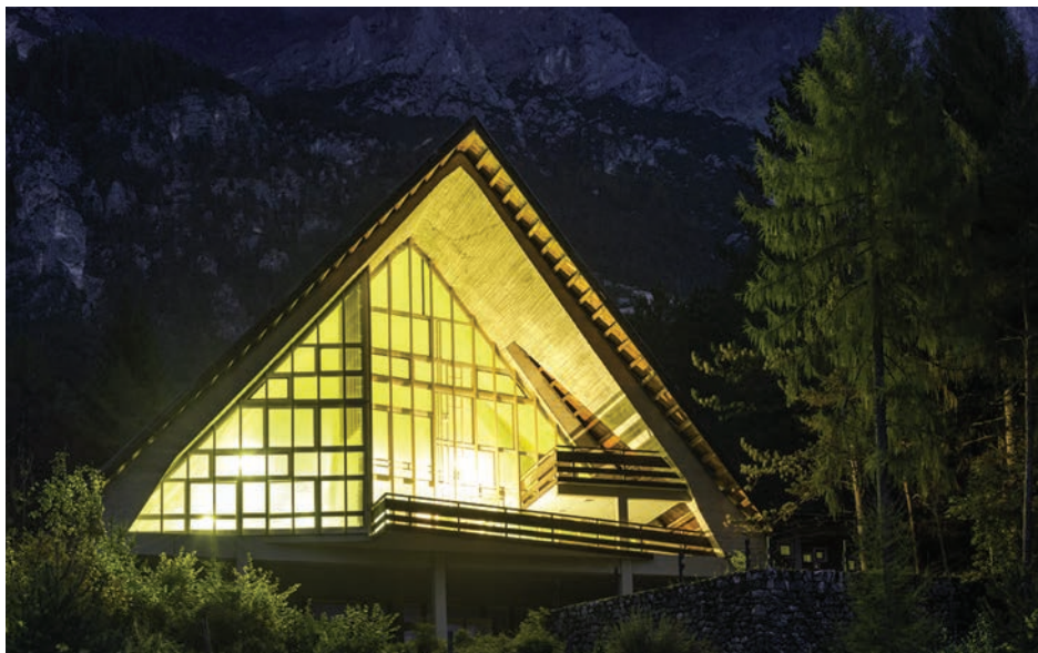
Fig. 5. Progettoborca , Public Hall (Aula Magna alla Colonia) at the former Eni Village summer-camp, designed by Edoardo Gellner, Borca di Cadore. Photo by Giacomo De Donà ©
