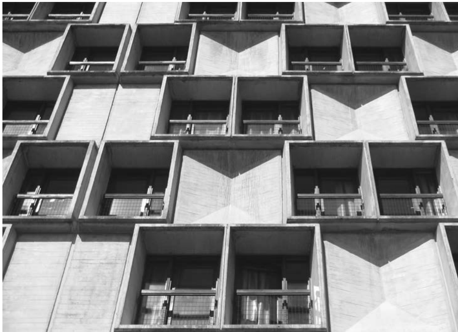
Fig. 10. Les Lindars hotel . Detail of the main facade
