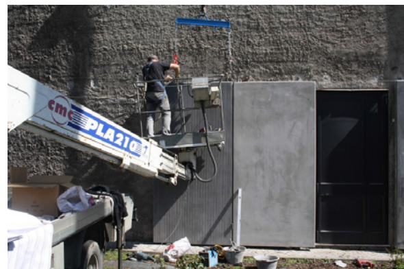
Fig. 11: Installation and levelling of the panels on the test façade.
