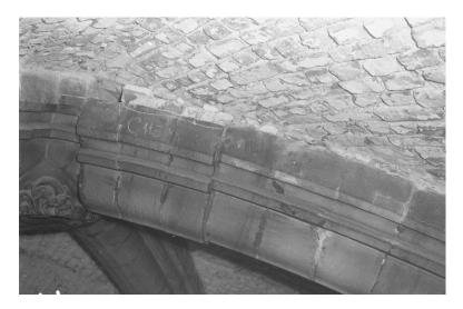
Figure 6. Sliding failure of a vault rib from Milan Cathedral (1965). Vault 113 in the plan in Figure 4.
