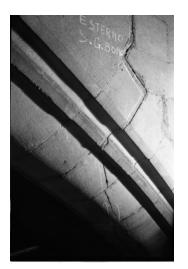
**Figure 3.** Shear/tension failure of masonry arch, Milan Cathedral (1965). At exterior arch from Pier 43 to Pier 44 on Figure 4.
