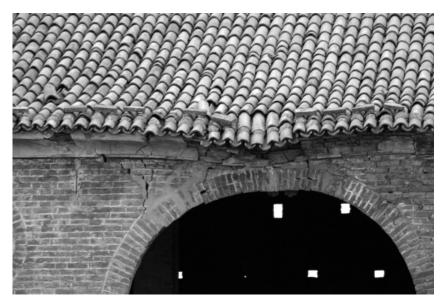
Figure 10. Sliding collapse of a brick arch.
