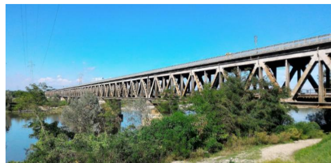
Figure 1 A photograph of the Bressana bridge taken from the railway access
