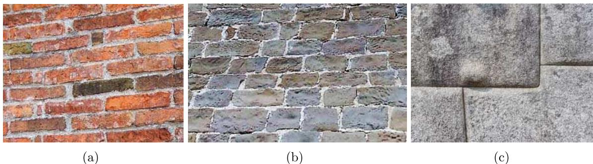
Figure 3: Examples of masonry: (a) brick masonry, (b) stone masonry and (c) Inca's masonry (dry stone masonry).
