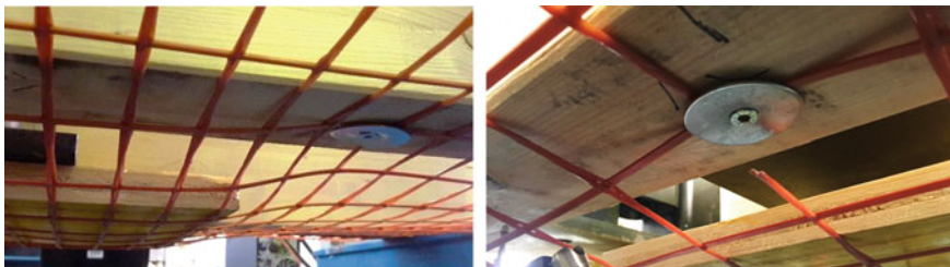
Fig. 8 Typical grid shear failure at anchor positions
