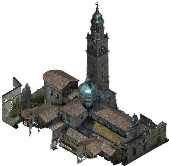
Figure 1: point-cloud of the complete digital survey for San Giovanni Evangelista church, Parma (courtesy of HeSuTech group).
