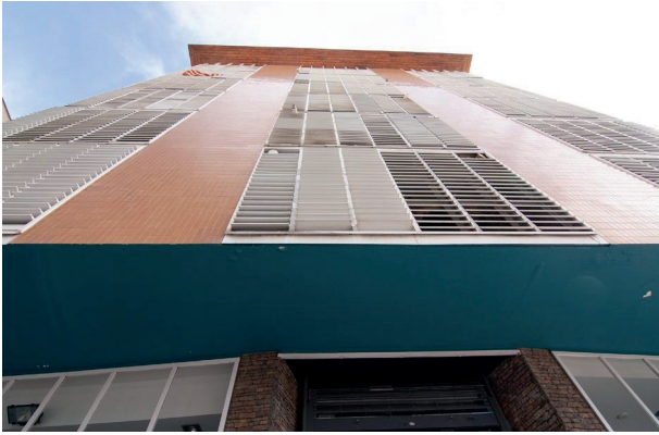
Fig. 6. J.A. Coderch, M. Valls. House ISM at Barceloneta (Source: M. Lucchini, 2017).
