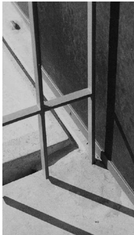
Detail of the parapet. Original picture. 8,8x14 cm (ACC 5.I/81 fotografie)
