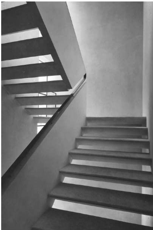
Interior staircase. Original picture, 1939. 17,3x12,3 cm (ACC 5.I/187 fotografie)
