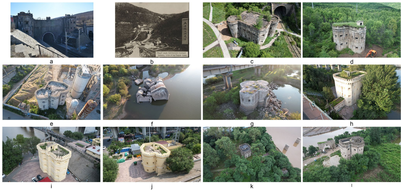
Fig. 5 Blockhouses of the key infrastructural elements along the CER Main Line: (a) Khing'an Range Tunnel Manzhouli-side blockhouse; (b) Khing'an Range Tunnel Harbin-side blockhouse (Anon 1919); (c) Xin'nangou Culvert along the Khing'an Range Loop Line Manzhouli-side blockhouse; (d) Xin'nangou Culvert along the Khing'an Range Loop Line Harbin-side blockhouse; (e) Nen River Bridge Manzhouli-side blockhouse; (f) Remains of the Nen River Bridge Harbin-side
