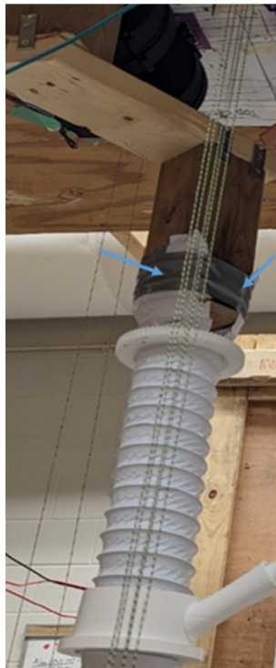
Fig. 116. Installing flexible tube onto 4x4 wood block support.
