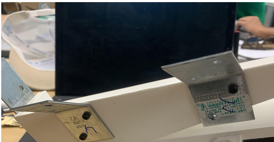
Fig. 100. Fastening L brackets to feeder enclosure.
