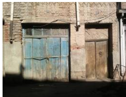
Fig. 18 Typical transom and decorative brickwork facade of a house in the neighborhood Barnava
