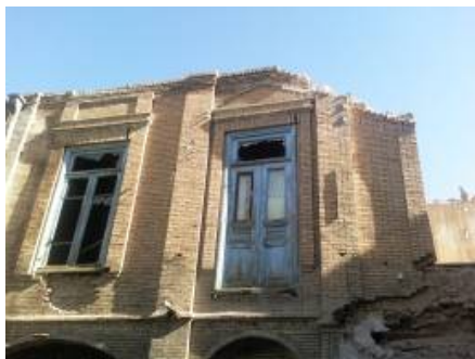
Fig. 17 Typical openings and decorative brickwork facade of a house in the neighborhood Barnava
