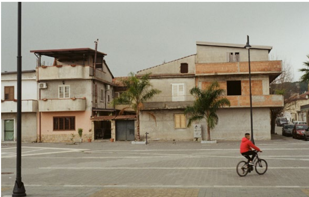
From the top, figure 20. Africo Nuovo, Reggio Calabria (photo N. Sulfaro, 2022); figure 21. Africo Nuovo in a frame from the movie "Anime nere", directed by Francesco Munzi, 2014.
