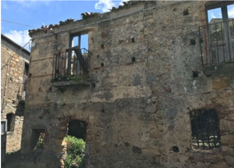
Figure 23. Ferruzzano, Reggio Calabria. The insertion of a portion built after the earthquake of 1908 on a pre-existing undamaged masonry (photo N. Sulfaro, 2022).
