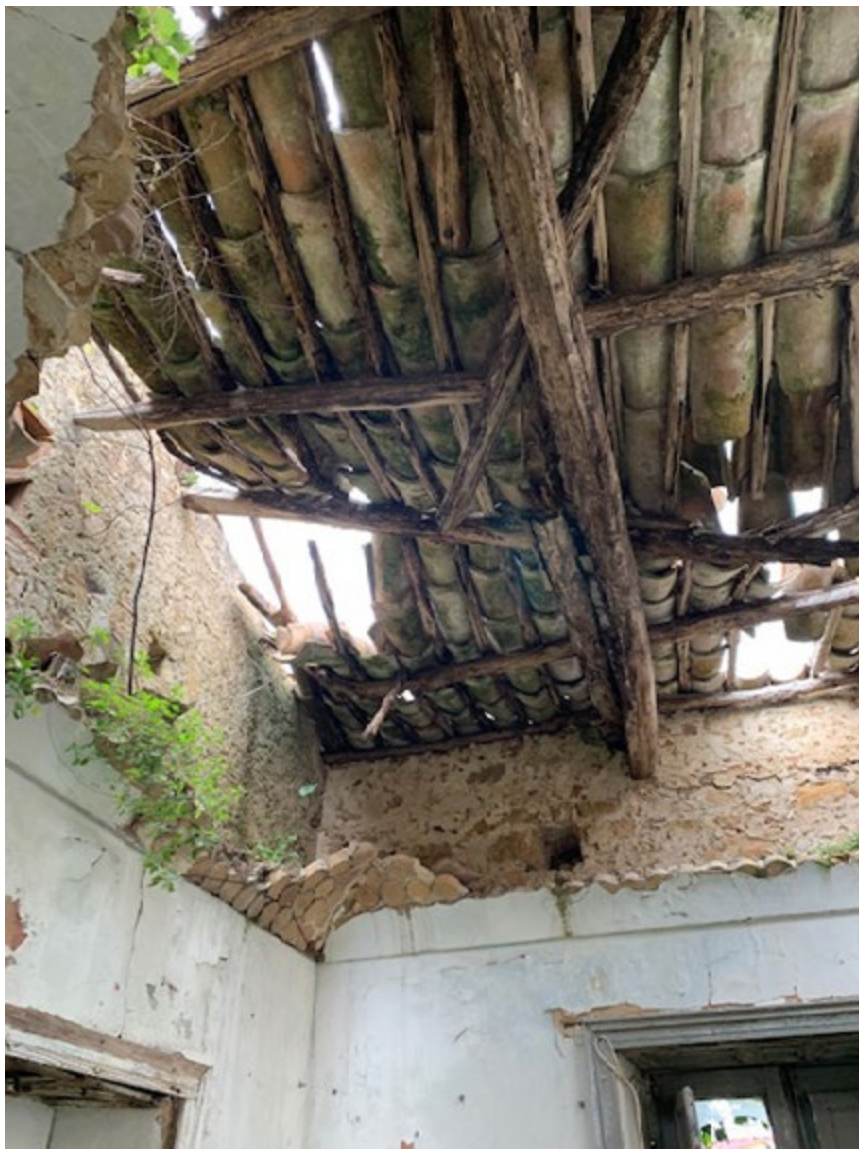
Figure 10. Ferruzzano Superiore. Traces of a vault made of carusi (photo C. Valiante, 2023).
