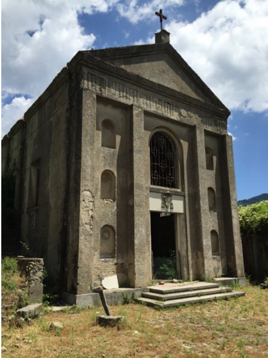
Figure 1. Africo Vecchio (Reggio Calabria). The church of San Nicola abandoned after the flood of 1951 (photo A.M. Oteri, 2023).
