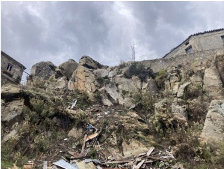
On the previous and on this page, figures 13-16. Ferruzzano, Reggio Calabria. The rocky outcrop where Ferruzzano is located shows a prevalent division according to vertical planes and prisms (photos N. Sulfaro, 2023).
