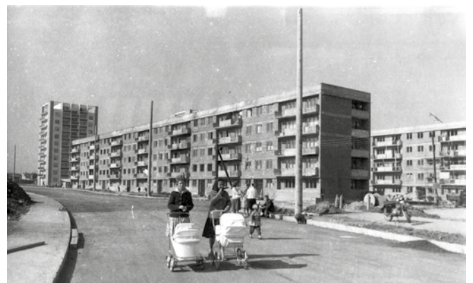
10 Construction site, microraión 1, Gheorgheni housing estate, Cluj. © N. Kulin, April 1965, DSAPC Cluj.
