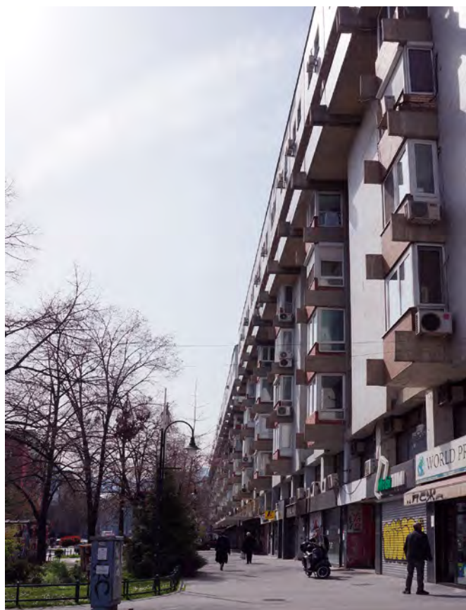
08 The pedestrian area along the City Wall housing complex, facing the inner-city ring road. © Vlatko P. Korobar, 2023
