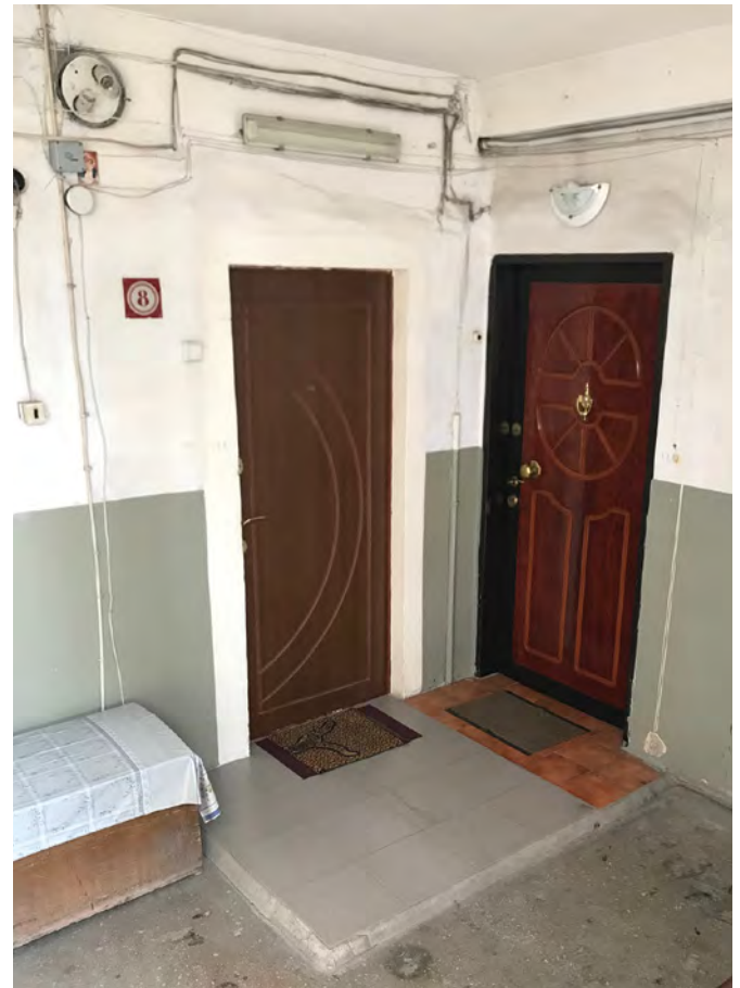
07 Small repairs and transformations of the shared entrance hall of a mass housing block (Yerevan) © M. Sapunova, 2022.
