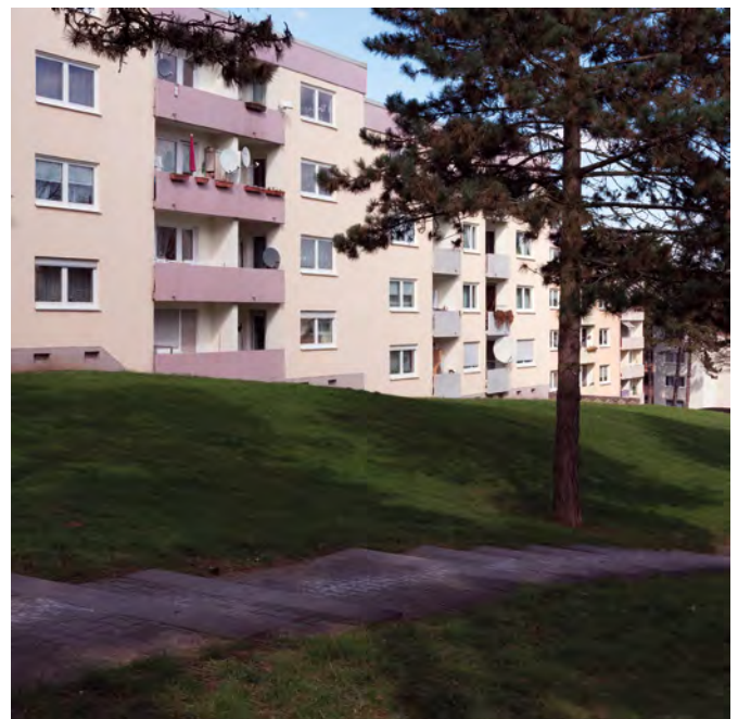
06 In Schelmengraben, buildings follow the slope of the landscape. © Malte Sanger, 2018.
