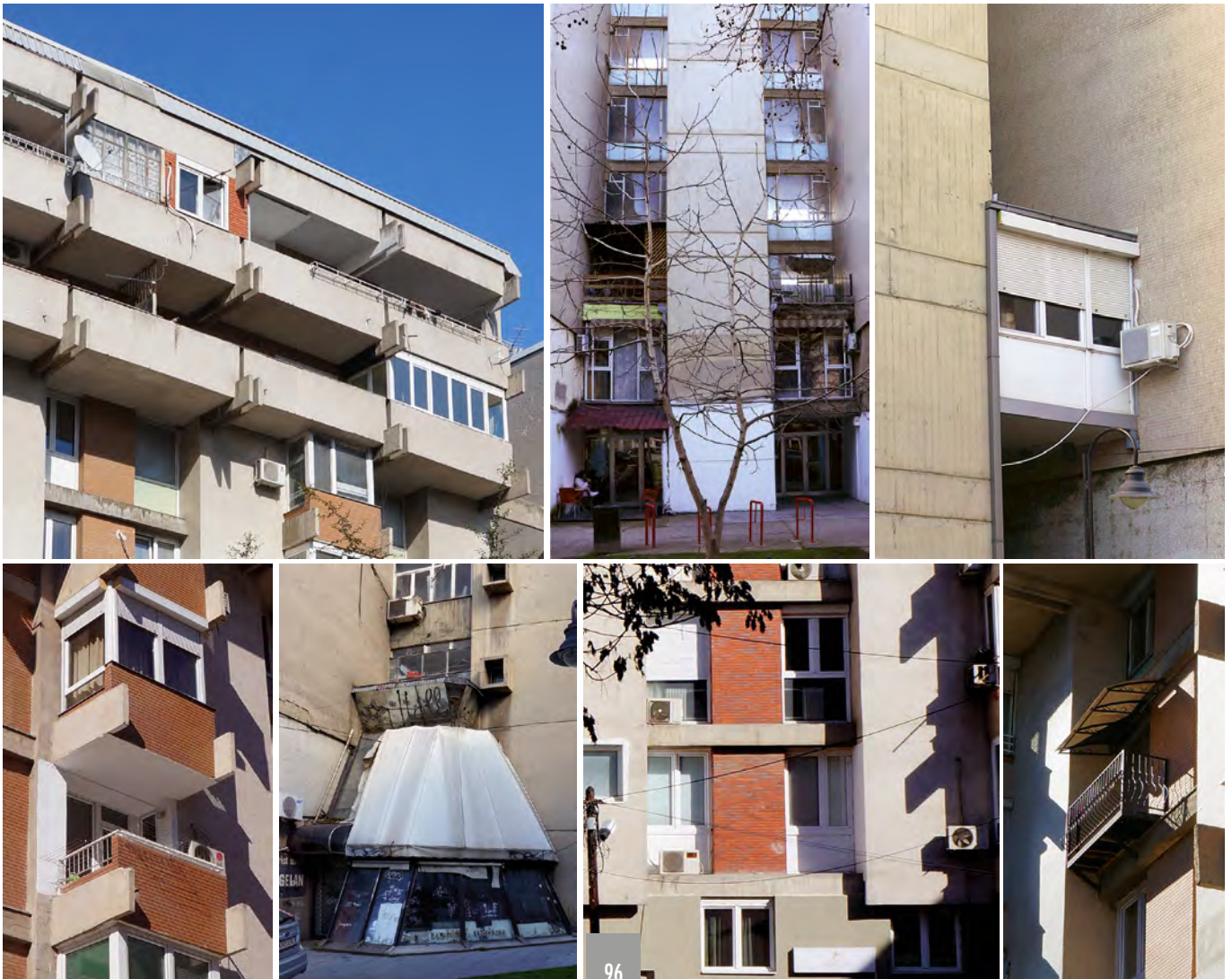
09 Alterations carried out by the dwellers, including sloped roof cover, enclosing parts of the terraces, adding new balconies, turning bay windows into balconies and other changes and additions to the facades © Vlatko P. Korobar, 2023.
