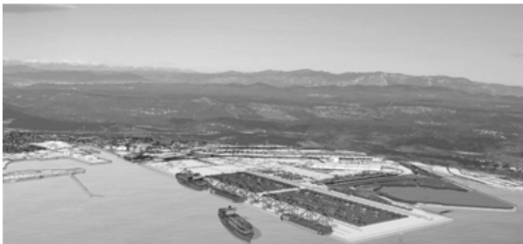
fig.6 - View of the Monfalcone Port Project
