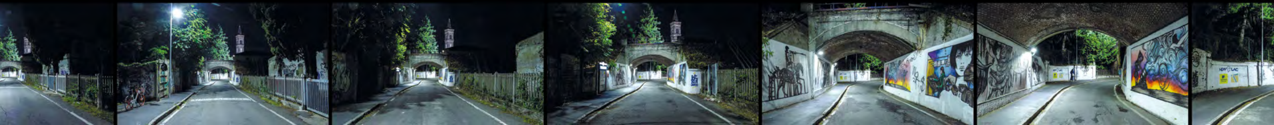
San Cristoforo Railway Underpass
