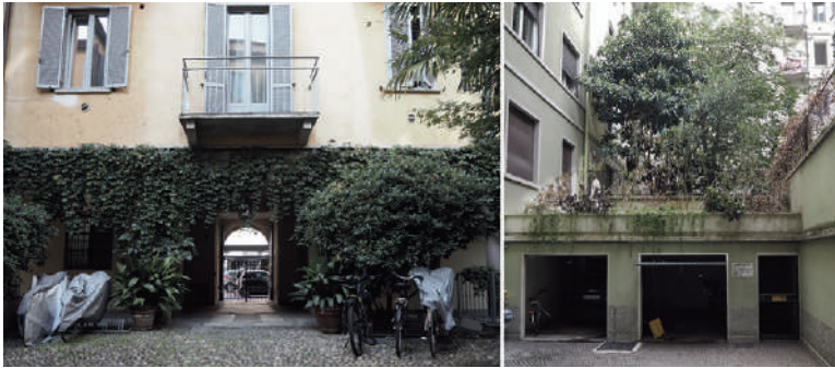
Fig. 7 | Horizontal and vertical green in the analysed courtyards, Milan, October 2021 (credit: M. S. Lux, 2021).
