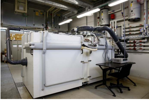
Figure 1: the DAVTB facility.
