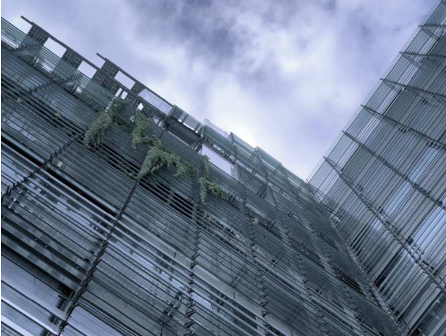
Fig. 1.2 Mario Cucinella Architects, SIEEB ( Sino-Italian ecological and energy efficient building ), Beijing. Façade systems examined as the external enclosing unit of the building organism, executed by means of the frameworks, made up of vertical and horizontal structural elements, in turn connected to the main load-bearing structures with interface devices, and by means of the “aggregative rules” for the assembly of the “pieces”, according to the component approach or componenting processes. © Courtesy of Mario Cucinella Architects
