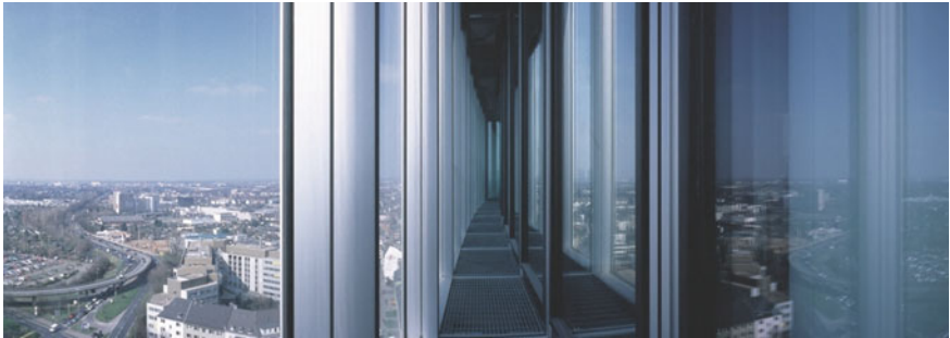
Fig. 6.17 Norman Foster and Partners with RKW (Rhode, Kellermann, Wawrowsky), Arag Tower , Düsseldorf. Functioning of the double envelope system which realizes the passive ventilation for cooling or heating of the internal spaces. © Courtesy of RKW
