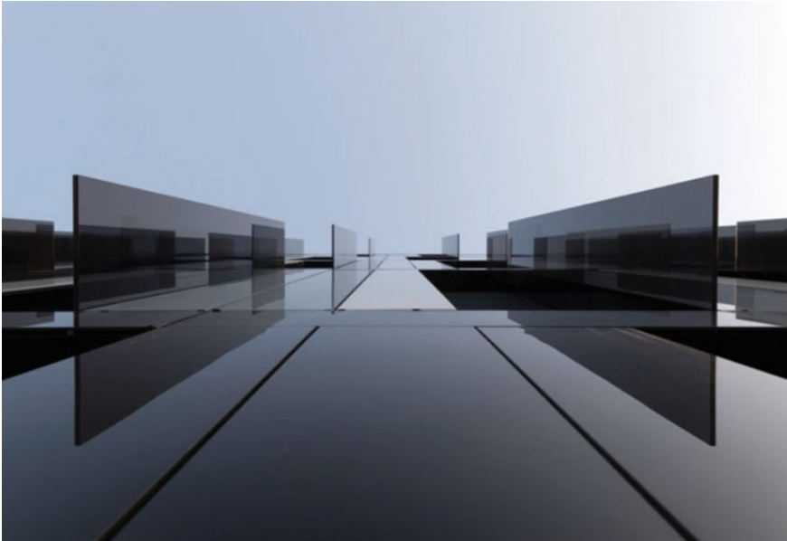
Fig. 1.11 Gianandrea Barreca and Giovanni La Varra, “B5” Building, RCS—Media Group Headquarters, Milan. Surface textures that take on the theme of the “barcode” rendered in a “dynamic” form through a cladding that alternates windowed parts with portions of the façade in screen-printed and coloured glass plates. © Courtesy of Focchi
