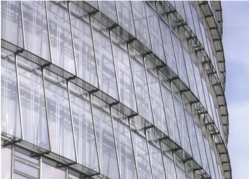
Fig. 6.8 Helmut Jahn, Post Tower , Bonn. Segmented external shading skin (south elevation), framed by linear vertical and horizontal aluminium profiles, that creates a visual and functional membrane to the internal curtain wall. © Courtesy of Helmut Jahn
