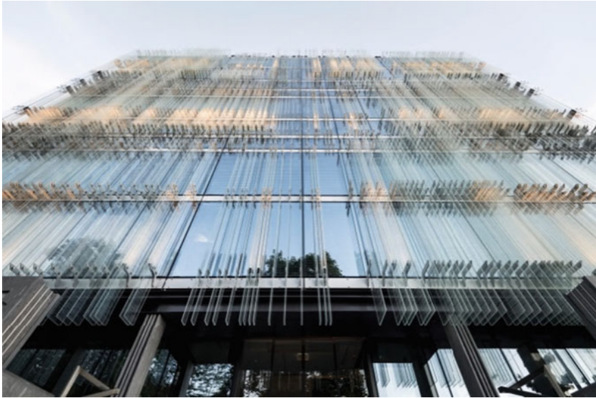
Fig. 1.13 Giovanni Vaccarini Architetti, Société Privée de Gérance (SPG) , Geneva. “Thick surface” of the envelope, with the help of screen-printed glass and protruding steel supports, proposed in a “volumetric” key: perceptive “dematerialization” of the vertical enclosures, established in a diaphanous and ethereal manner, sensitive to the luminous and chromatic variations of the surrounding environment. © Courtesy of Alex Filz
