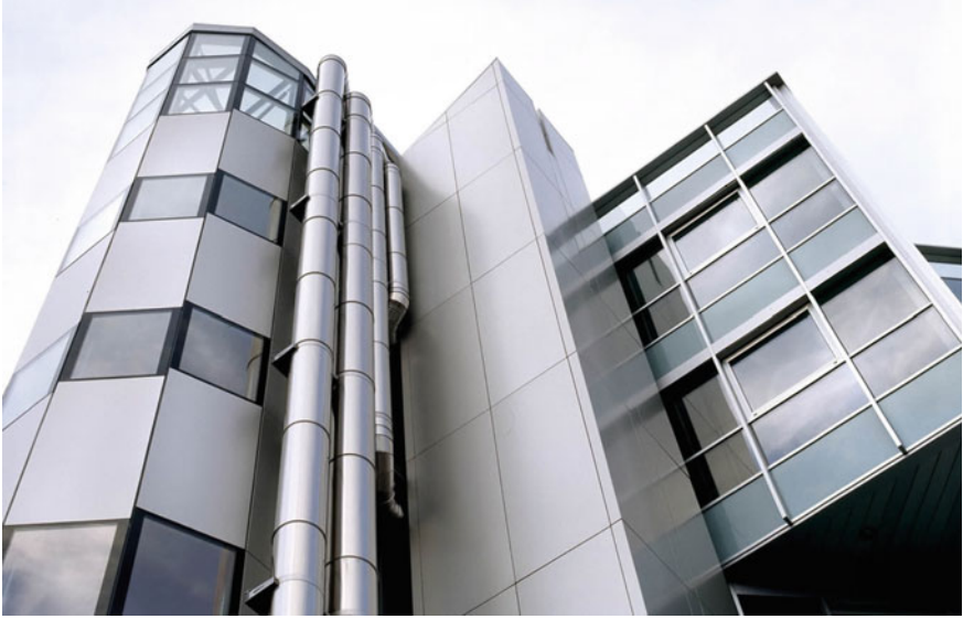
Fig. 3.1 Lotti Architetti, Ascom Office and Trade Building , Pistoia. Procedures for aligning façade modules in the absence of external profiles, using structural silicone support frames for transparent and opaque closures. © Courtesy of Schüco
