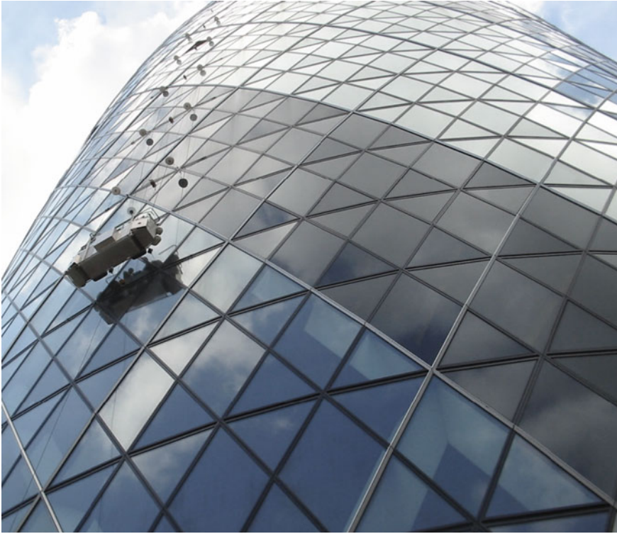
Fig. 6.2 Norman Foster and Partners, Swiss Re Tower, London. Type of enclosure enveloping the cylindrical tower, streamlined and tapered according to a progressive double-curved conical winding (double-curved geometry). The closure, warped by the diagonal lattice construction, is composed of the double envelope system that generates an upward air flow (stimulated by the “chimney effect” and increased by the thermal gradient between the temperature in the cavity and the temperature of the incoming air). © By the Authors
