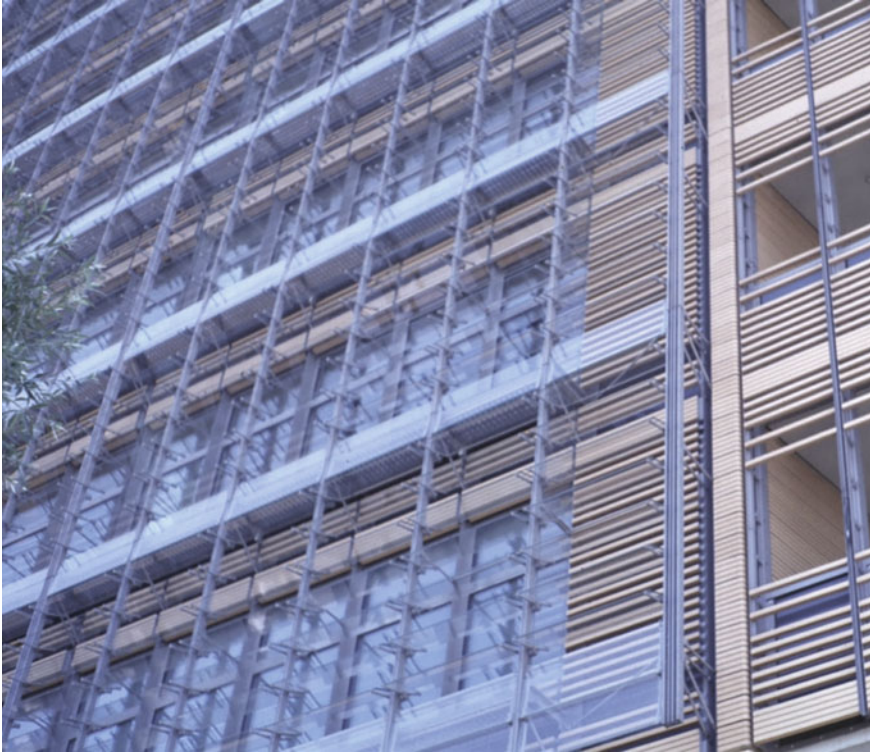
Fig. 6.1 Renzo Piano Building Workshop, Debis-C1 Building, Potsdamer Platz sector, Berlin. Functional and environmental expression of the façade components: the outer membranes made of glass sheets create, when closed, a thermal and sound-absorbing storage cavity and, when open and regulated, a filtering function with respect to incident wind loads. © By the Authors
