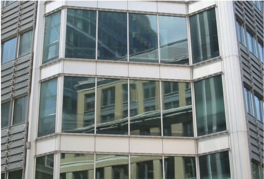
Fig. 2.2 Nicholas Grimshaw and Partners, Building in 25 Gresham Street, London. Construction of the mullions and transoms façade system according to the interposition of the horizontal spandrel panels between each level of the curtain. © By the Authors
