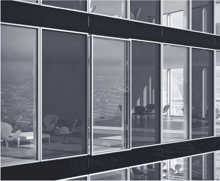
Fig. 1.9 Energy System. “Specialized” and calibrated elaboration of the envelope with respect to the fine-tuning of the “organic” devices integrated with external stresses and the plant engineering apparatus, in the form of the interfaces of interaction, mediation and interchange with climatic actions © Courtesy of Schüco
