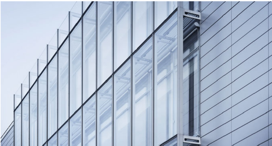
Fig. 6.6 Maurizio Varratta, iGuzzini Lab , Recanati. Assembly of the external screen, in the form of a totally or partially transparent façade, made up of monolithic tempered or double-glazed glass panes. © Courtesy of Pichler Projects
