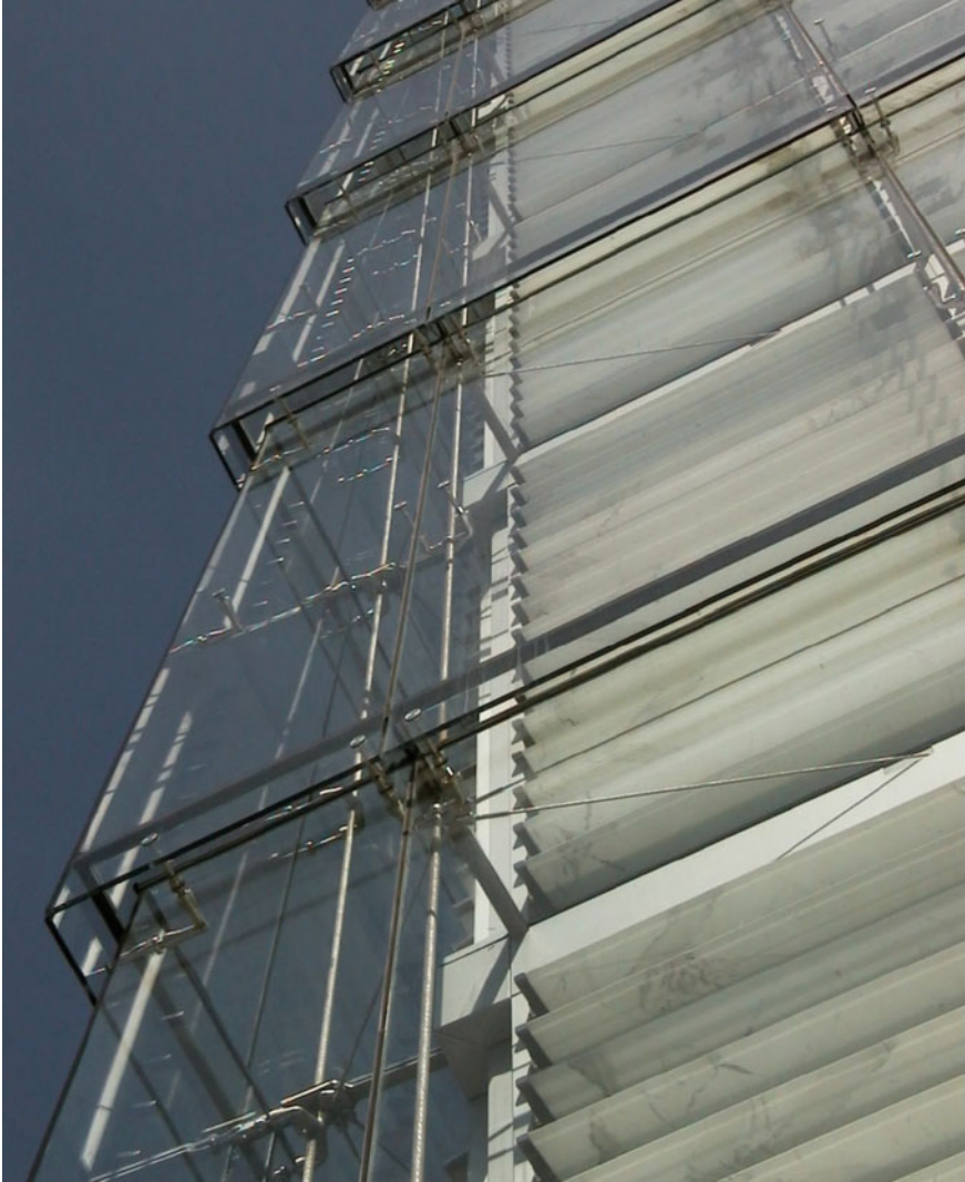
Fig. 1.4 Jim Clemes, Centre Royale Monterrey , Luxembourg City. Envelope components arranged in an “integrated” form according to the processes of “specialization”, in accordance with the configuration of the layers of materials, composed of or resulting from the assembly of multiple elements, and the processes of “aggregation” between functional apparatuses. © Courtesy of Bertl
