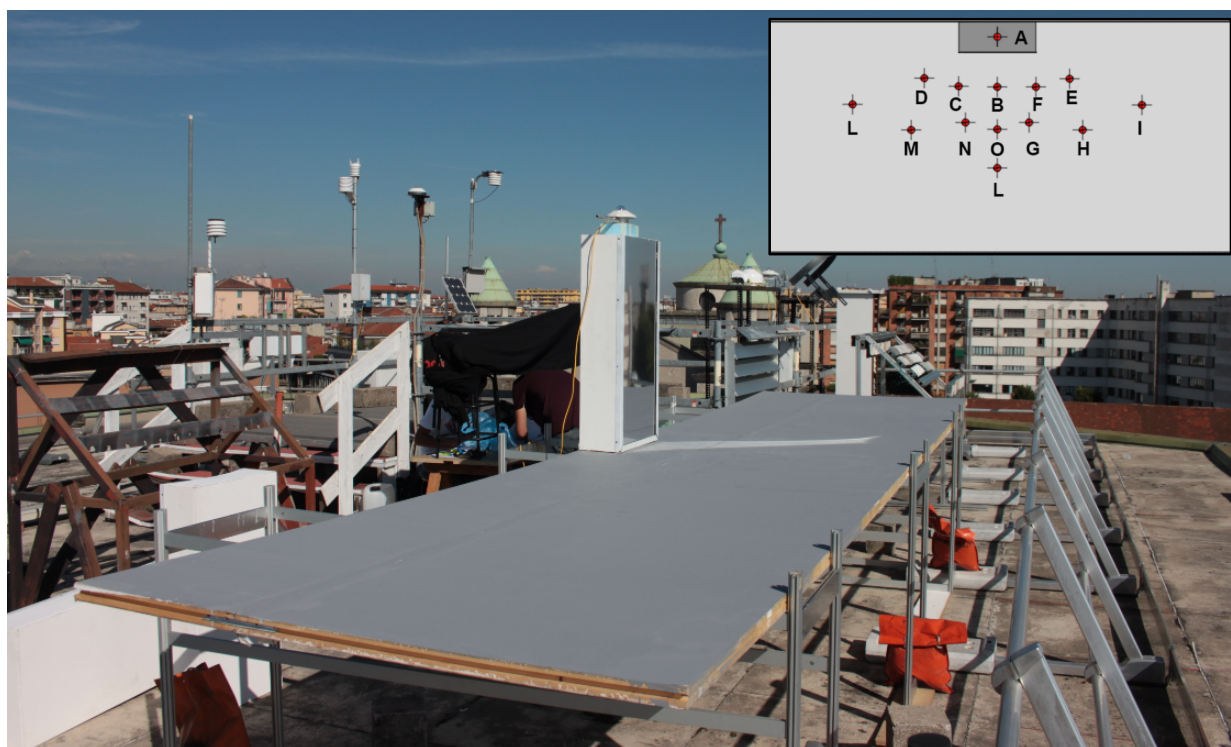
Figure A2. Flat reflective façade—Experimental setup and measurement points position (Figure 2).
