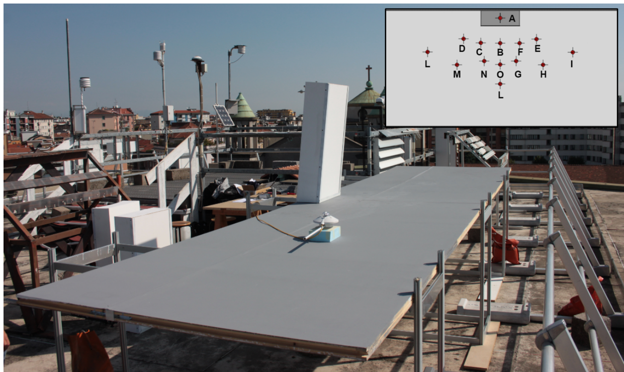
Figure A3. Flat 10% tilted diffusive façade—Experimental setup and measurement points position (Figure 2).
