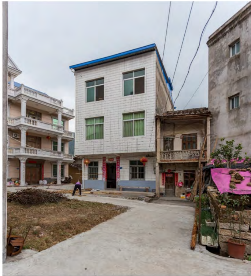
Figure 8. Problematic formal and material juxtapositions. Picture by the author, November 2017.
