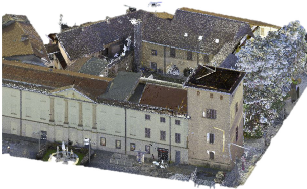
Figure 1: View of point cloud generated from the laser scanner survey
