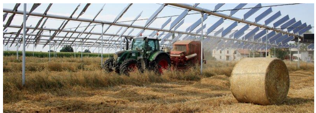
Figure 16. View of the dual use of land with the PV track system on the upper layer and agricultural works at ground level (photo: © REM).
