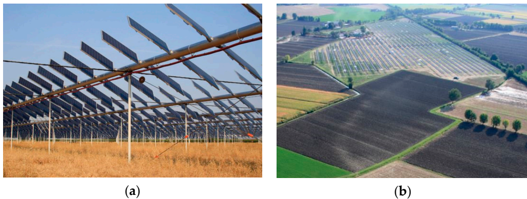
Figure 17. (a) View of the PV track system during the first crop (photo: © REM); (b) aerial view of the solar plant in landscape (photo: © REM).
