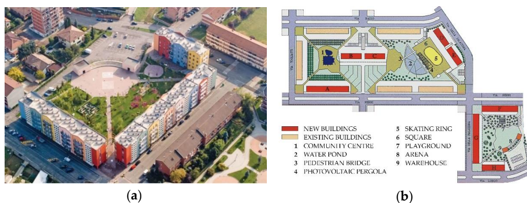
Figure 4. The (a) aerial view of new buildings in the eastern part of the Photovoltaic Village (source: © Municipality of Alessandria) and a site plan of the entire area indicating the position of facilities, new and existing buildings (b) (source: © Municipality of Alessandria).
