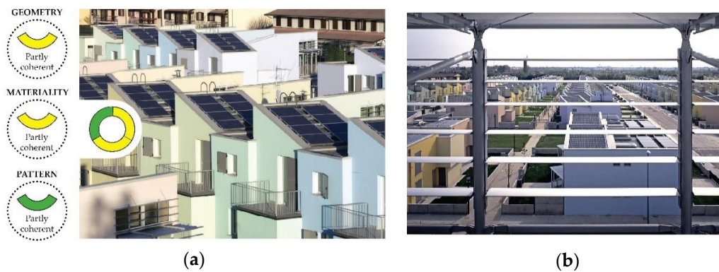
Figure 12. Architectural integration matrix for the PV systems at Violino District in Brescia (left); (a) system modular pattern (photo: © Fabio Cattabiani); (b) view from the roof of one of the multi-family houses (photo: © Fabio Cattabiani).
