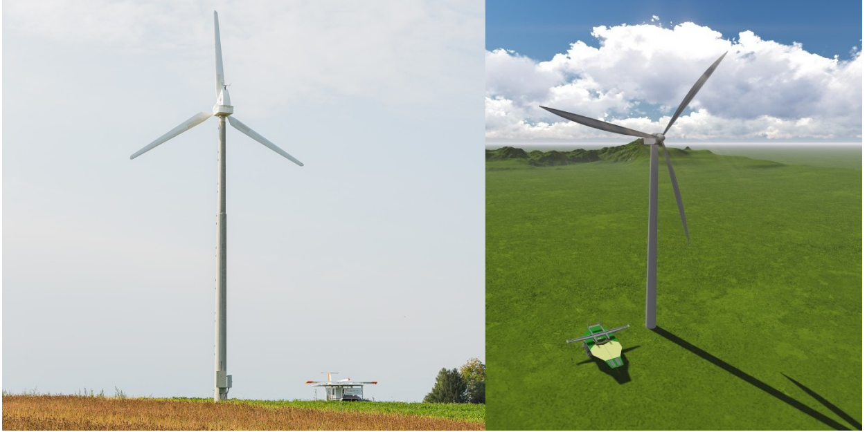
Figure 3: Conventional wind turbines next to docked AWE systems of comparable rated power: photo of the TwingTec pilot system [35] (left) and rendering of the envisioned offshore system of Ampyx Power, the AP4, with a rated power of 2 MW [36] (right).
