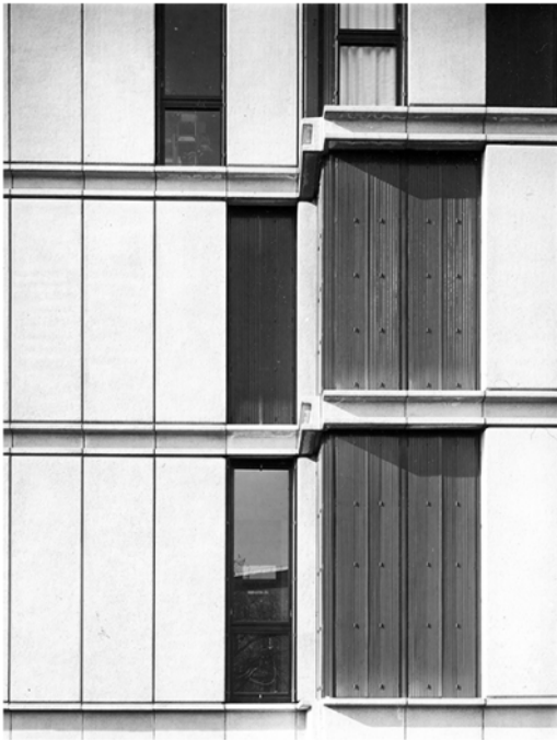
Figure 5. Prefabricated panels of façades (Archive Angelo Mangiarotti, Milano).
