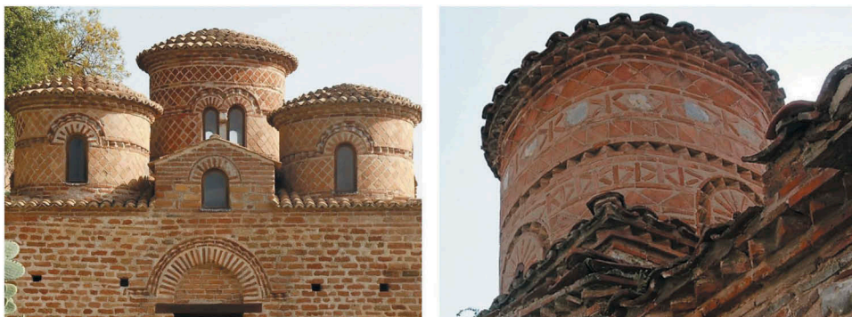
Figure 7. The lozenge decoration motive on the domes of the Cattolica di Stilo (left) and the dome of the 10th century church of Panagia Koumbelidiki in Kastorià (right).
