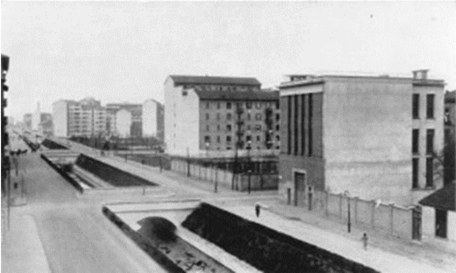
Fig. 3. The first phase of the reconstruction of the Olona riverbed until its filling, 1930s. Source: author's archive.
