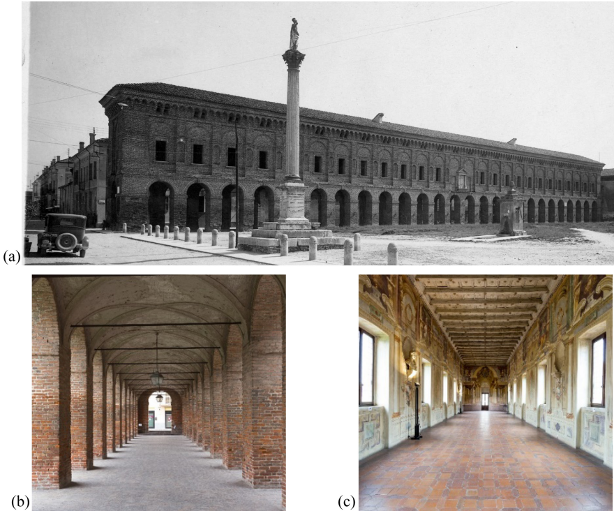
Fig. 1. Historic view of Galleria degli Antichi (a), masonry columns and crossed vaults (b), and first-floor level of the construction with the lacunar ceiling (c).
