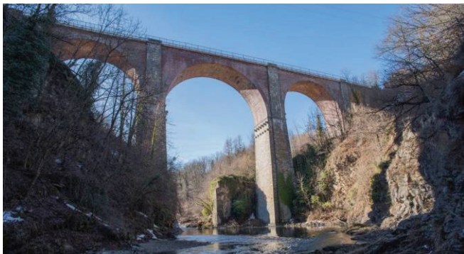
Figure 1. The Olla bridge, view from the Stura river.
