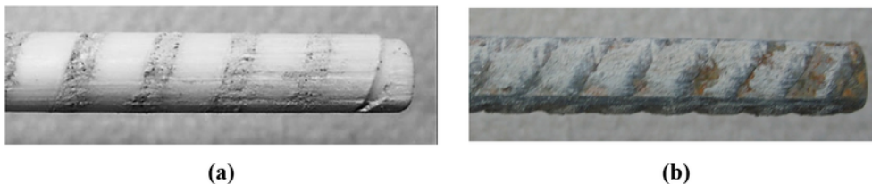
Fig. 11. Surface of (a) GFRP and (b) steel bar of diameter 8 mm, concrete C4 and cover 10 mm, after pull-out.
