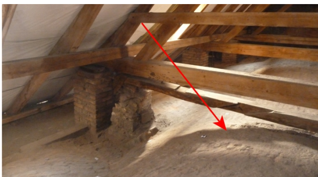
Figure 8. The arch built at the end of the first construction phase
