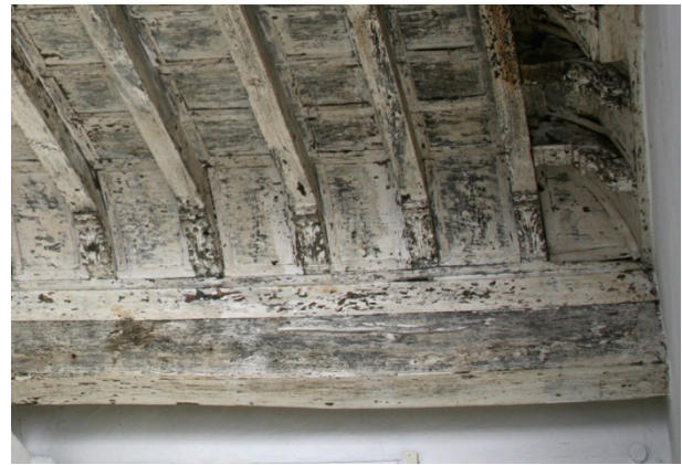
Figure 10: Floor with bussole covering joists and corbels from the late 15 th century (Palazzo Affaitati-Soldi).
