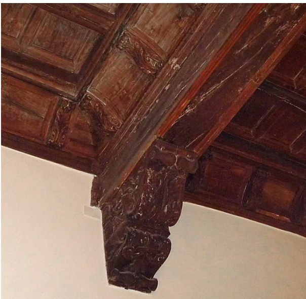
Figure 5: Detail of the floor in fig. 4.
