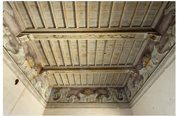
Figure 6: Timber floor with old girders; joists and planking were renewed between the late 17 th and the early 18 th centuries.
