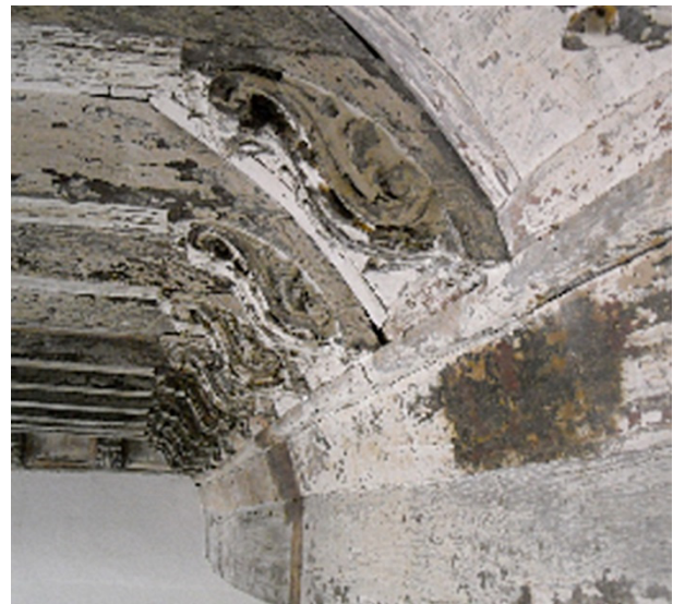
Figure 11: Detail of the floor in Fig. 9.
