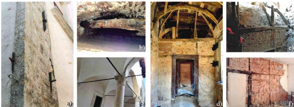
Figure 7: Anti-seismic measures adopted in Carli Benedetti Palace in L'Aquila: a) heads of the metal tie rods connecting vertical walls to horizontal structures; b) timber (radiciamento) reinforcing a masonry wall, connected to a metal tie rods crossing a chimney flow; c) tie rods at the intrados of the arches of the porch; d) the 18 th century additions composed by wooden frames, directly connected to e) the wooden reinforcements of the vaults, forming a box-like devise with f) the vertical partitions (pictures from [15] elaborated by the authors).
