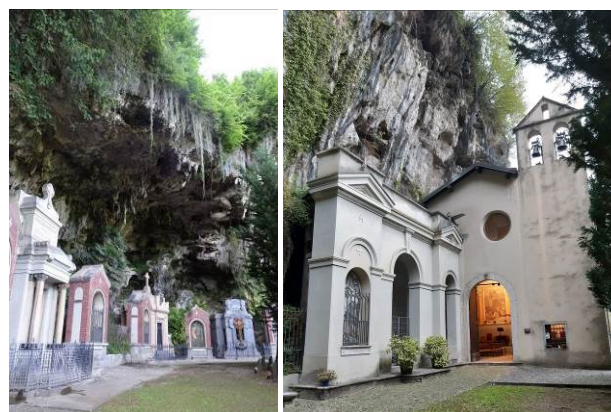
Figure 1. The Laorca monumental complex (the Via Crucis on the left, and the "San Giovanni ai Morti" church on the right).
