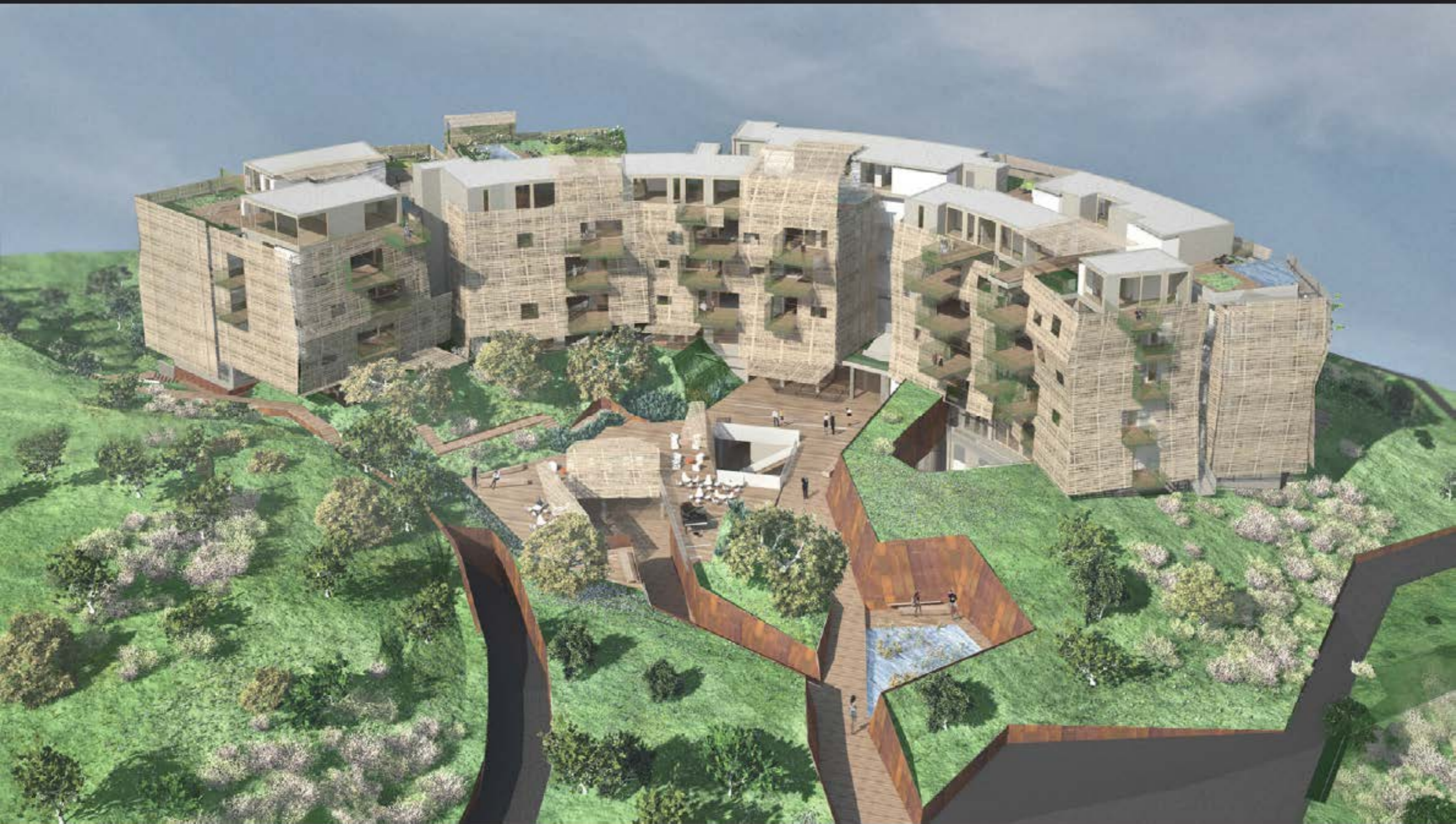
south-west general view
