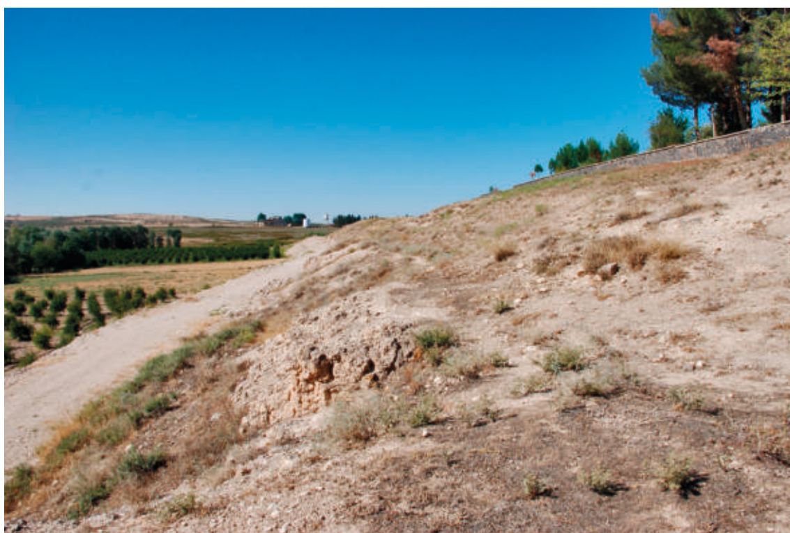
2. General view of the North-South Slope from East.
