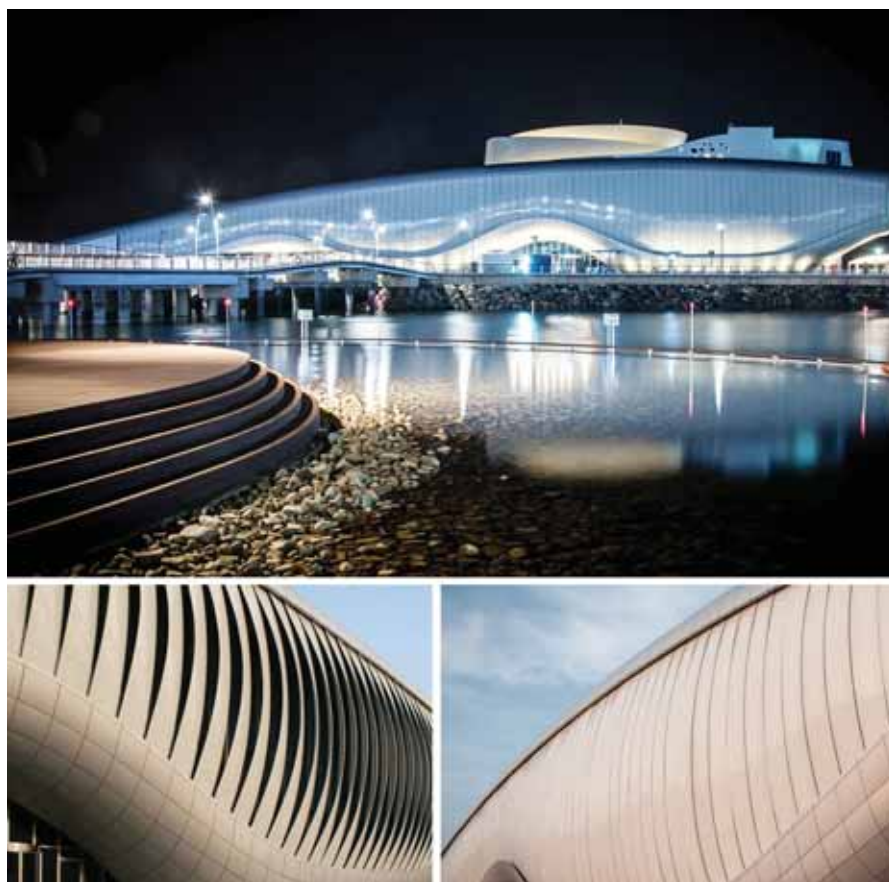
Fig. 4.4 - Soma Studio. Thematic Pavilion for Yeosu Expo 2012 (©Soma). The design's concept for the 140 meters long and 3 to 13 meters height dynamic façade originated from biology and is an example of a central level system. The 108 kinetic lamellas controlled internal light conditions and created organic external animated patterns. Servomotors reduced the distance between the two bearings to originate the movement, resulting in a side rotation of the lamellas.
