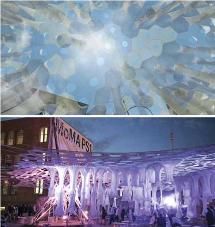
Fig. 4.5 - Jenny Sabin Studio. Lumen, New York (© Jenny Sabin Studio). Lumen consisted of 250 hanging tubular structures designed to capture and react to changes in sunlight over the day. The concept originated from biology, and its composition refers to a local-level systems typology. The structure's reactive surface was linked to human interaction and environment.
