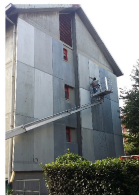
d) Positioning of the covering panels with crane
