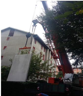
a) Panel's lifting by crane
