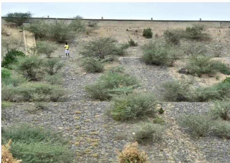
Figure 5: the view of the dam (photo 2014).
