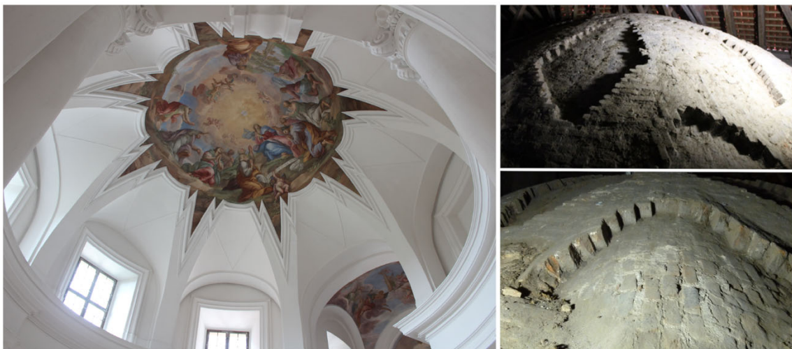
Fig. 2 St. Bernard's chapel. Left: Vault intrados: eight lunettes and ribs, central frescos by artist J. A. Pink. Top right: vault extrados: Y-shaped ribs with interlocking bricks on the two edge of the lunettes. Bottom right: lunettes brick arrangement
