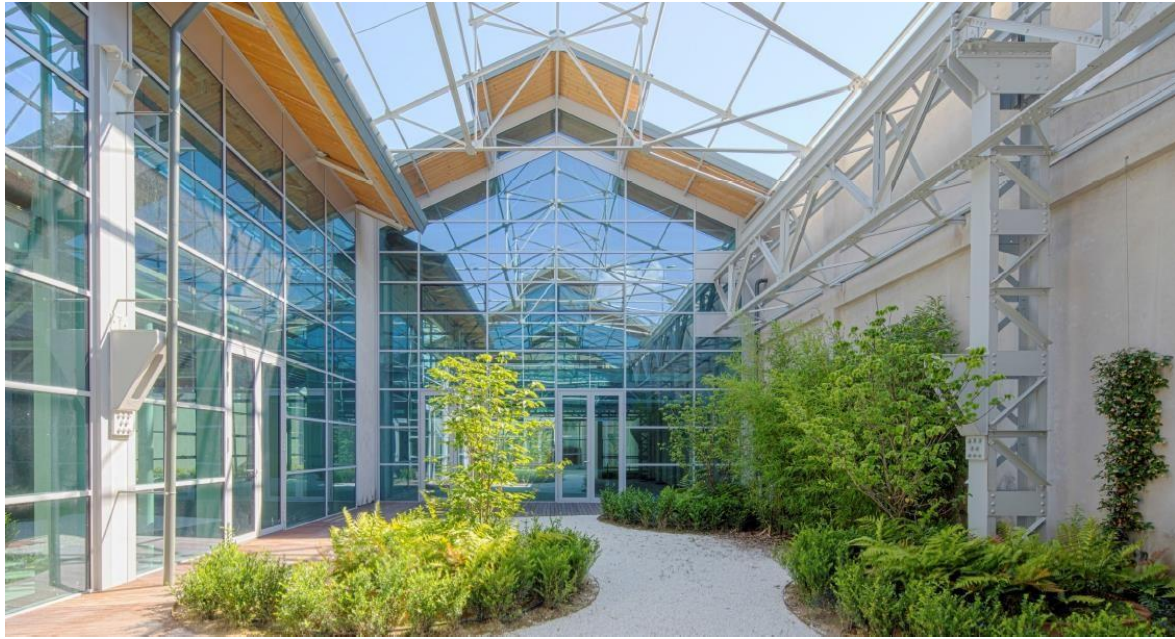
Fig. 6: The Tempra building. The original metallic structure were preserved in this building
