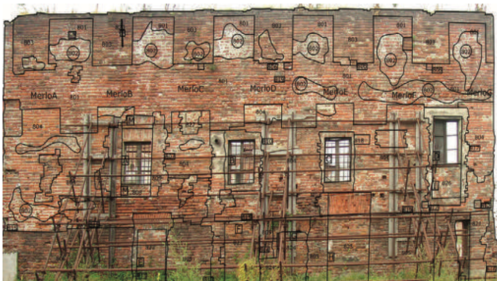
Fig. 7 | Stratigraphic survey of the western facade of the wall (credit: Albani, Gambaro and Mittermair, 2005).
