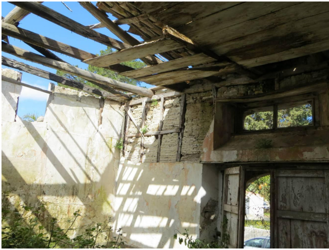
Fig. 5. Timber-frame structure of the Bishop's Palace at Mileto. (Image by Nicola Ruggieri.)
