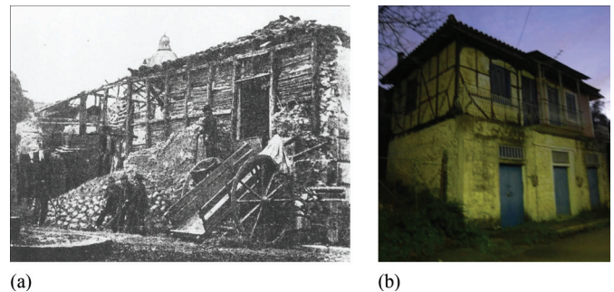
Fig. 2. (a) Borbone structural type. The damage caused by the 1908 earthquake was due to the stone structure and poor material properties, which favored the wall overturning; the timber frame suffered limited damage (reprinted from Commissione Genio Civile 1909); and (b) the traditional Lefkada type, with stone masonry at ground level and a timber frame at the first story (image by Sandra Tonna).
