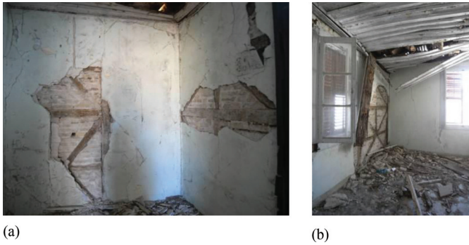
Fig. 8. Internal views of timber-frame organization on the first floor: (a) the horizontal, vertical and diagonal elements distribution in the vicinity of a corner; and (b) the panel organization near an opening. (Images by Sandra Tonna.)
