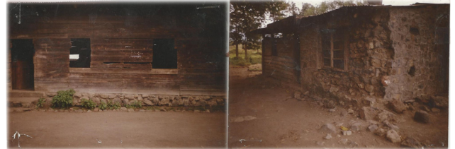
Figure 1 - Ngarenanyuki School in 2003 (dilapidated wood and soil building).
