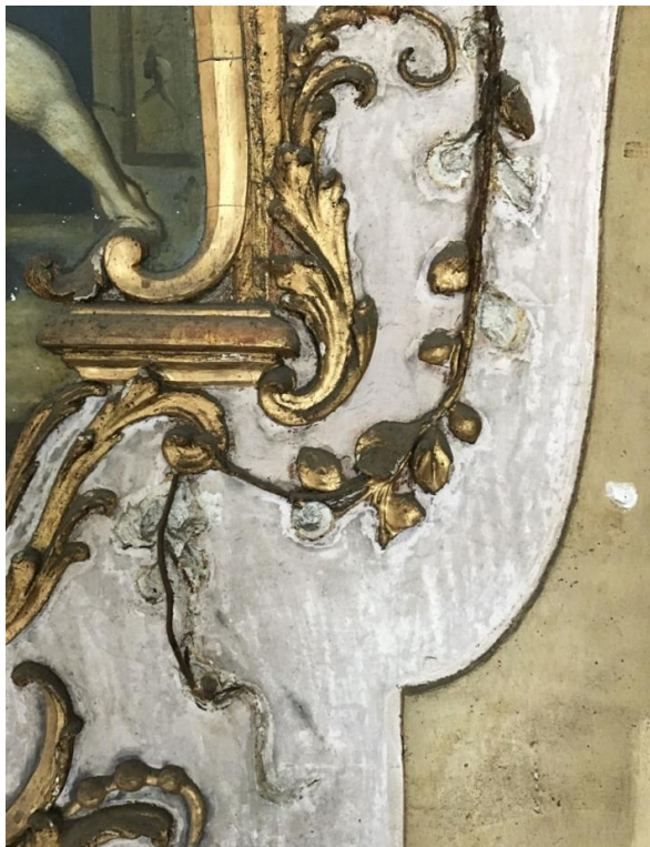
Figure 11. Wall 2: detail of the iron wires resembling stems from which leaves and blossoms hang.
