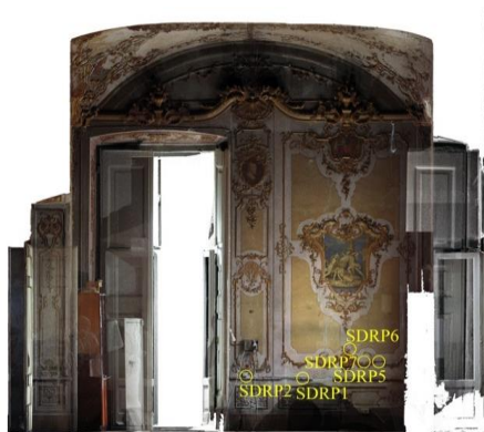
Figure 6. Laser scanner survey of the Gabinetto of gilded stucco. Wall 2 with sampling points.
